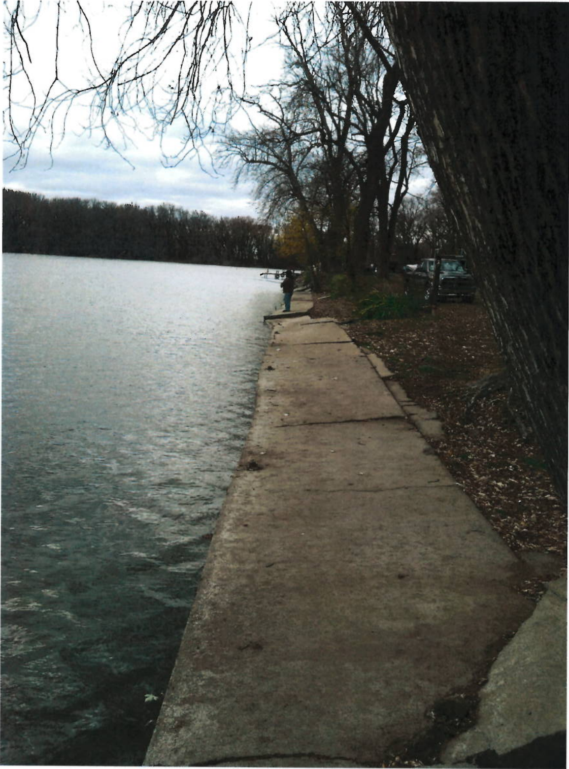
View of Sea wall from the North looking South:
