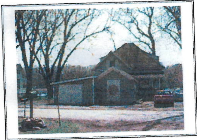
REAR OF SUBJECT PROPERTY (Street Side)
