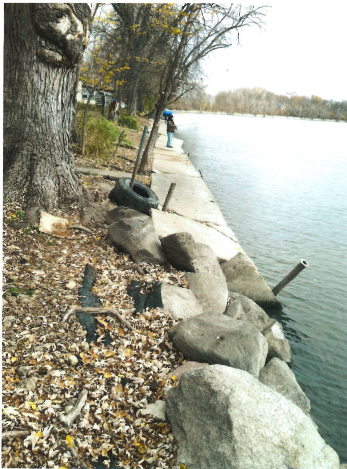
View of seawall from the South looking North:
